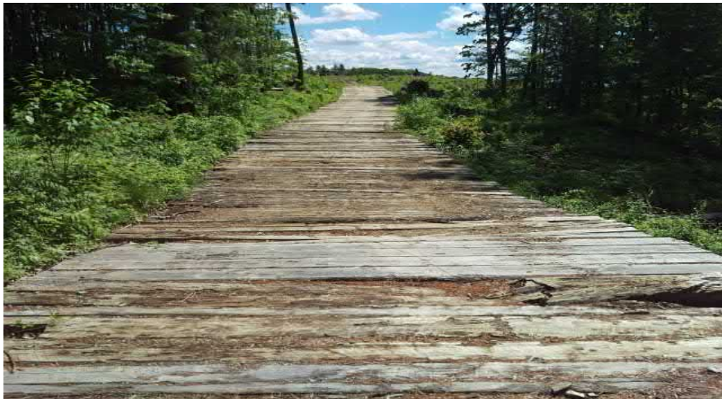
View of construction entrance timber mats — facing south
