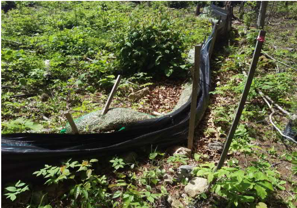
View of damaged silt fence in northern portion of the Site — facing north
