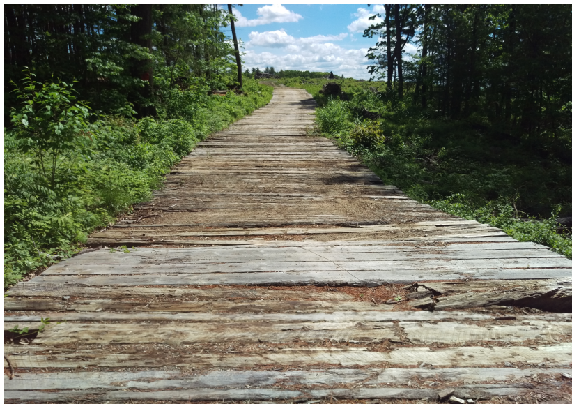
View of construction entrance timber mats — facing south
