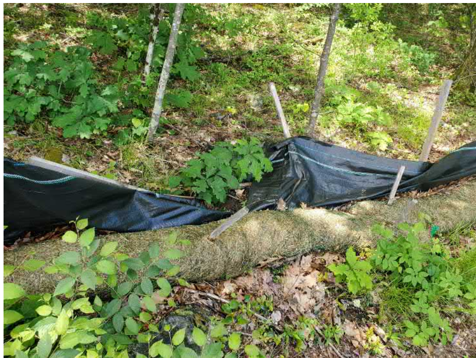
View of damaged silt fence in southeast portion of the Site — facing southeast
