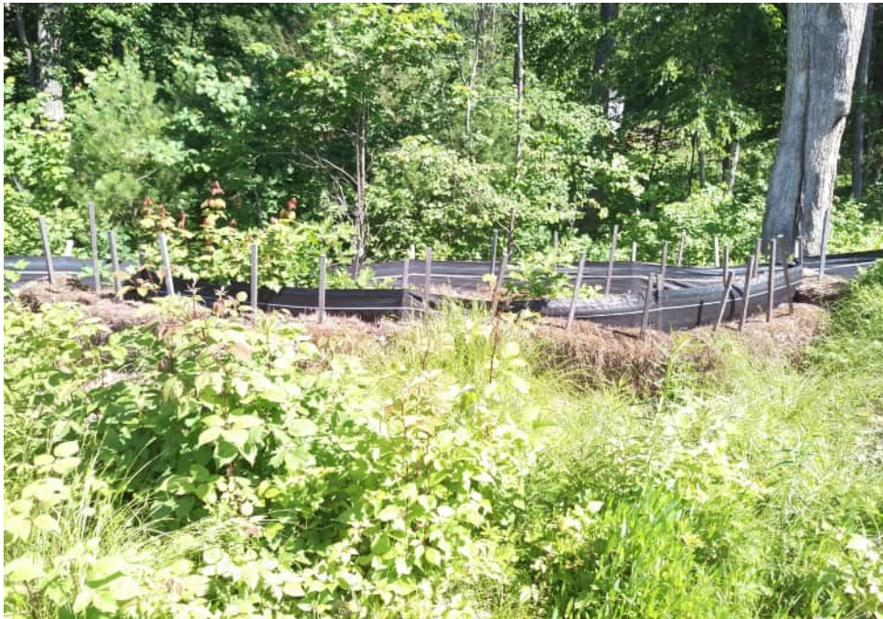
View of haybales and silt fence in northern portion of the Site — facing north
