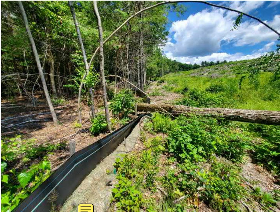
View of fallen tree damaged to silt fence in southwestern portion of the Site — facing north
