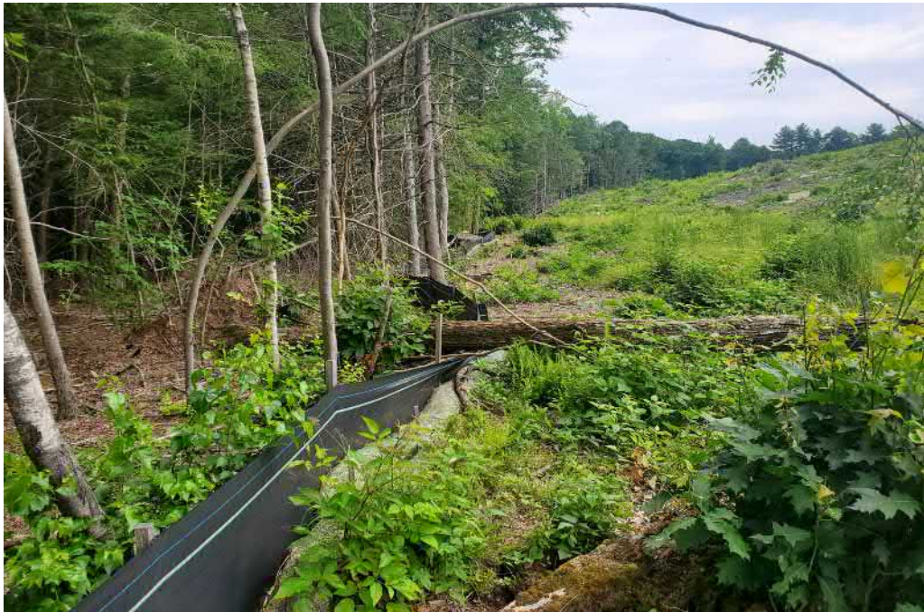
View of fallen tree damage to silt fence in southwestern portion of the Site — facing north
