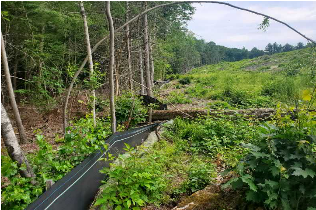
View of fallen tree damaged to silt fence in southwestern portion of the Site — facing north
