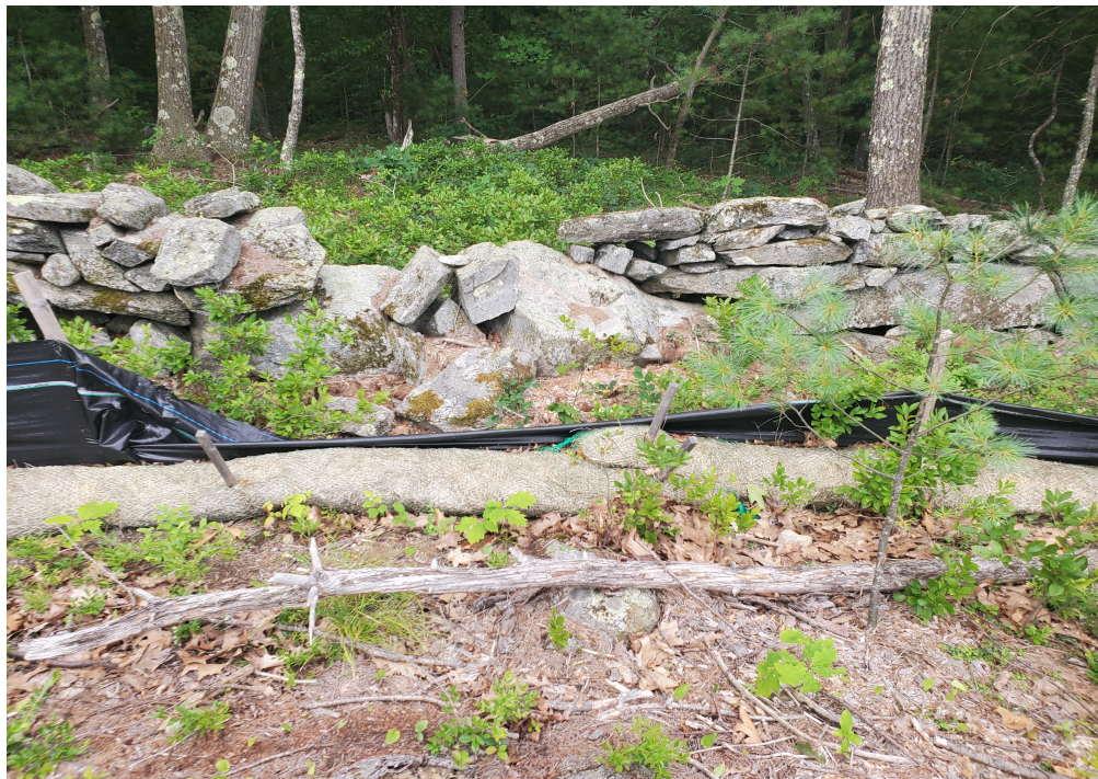
View of damaged silt fence in northeastern portion of the Site — facing east
