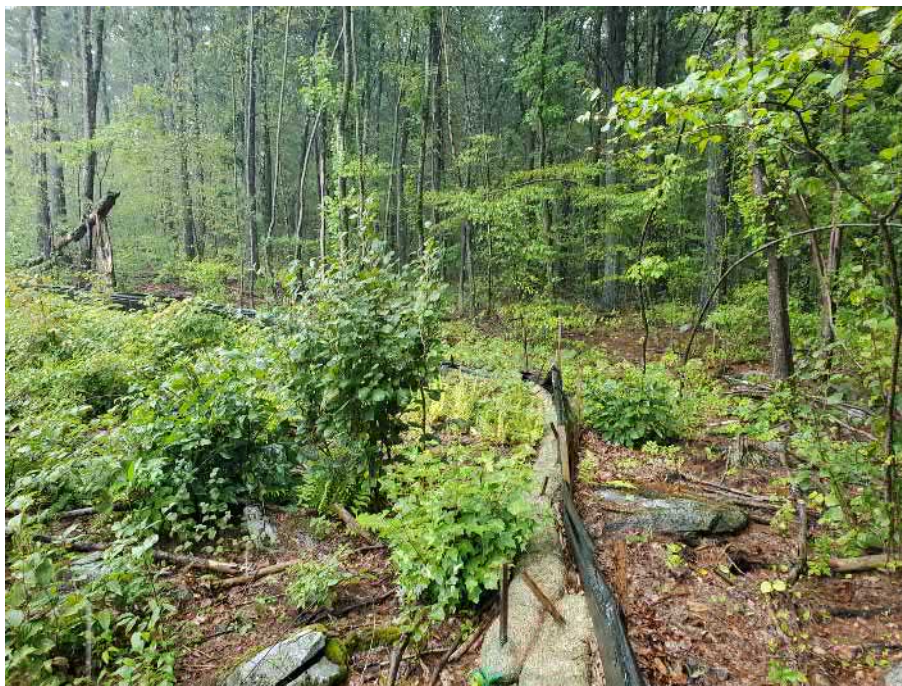
View of damaged silt fence in northeastern portion of the Site — facing east
