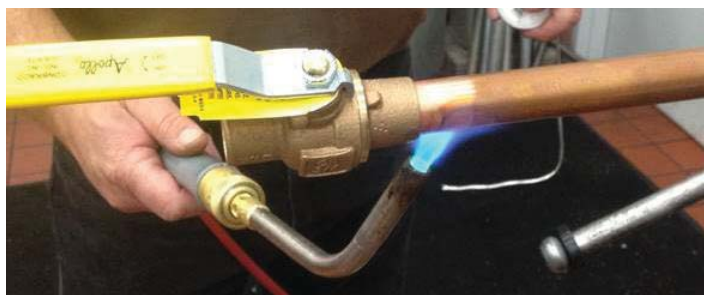
Figure 1 - Preheat tubing
