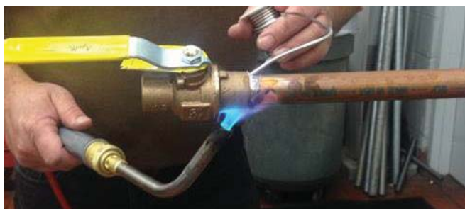
Figure 2 – Heat valve cup area and apply solder
