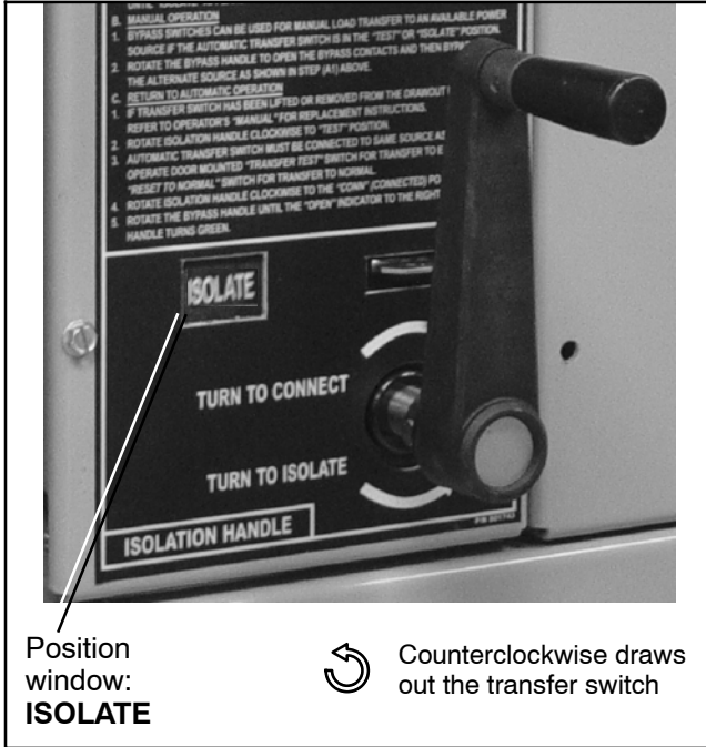
Figure 7-17 Isolation Handle Turned to ISOLATE.
