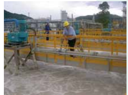
5 HYPERCLASSIC® -Mixing & Aeration Systems in an industrial wwtpt in Brazil (Chemical Industry)
