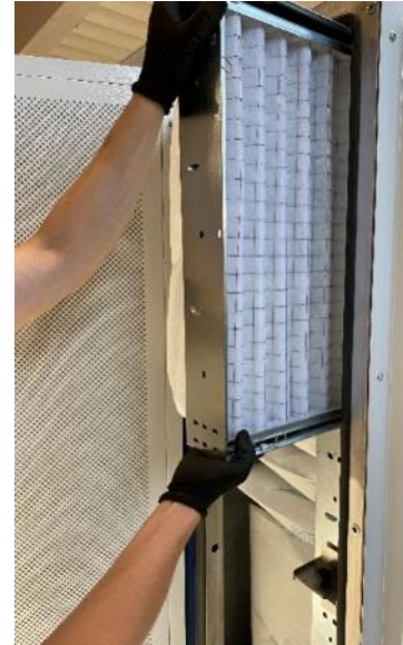
Pull-out the filter frame
