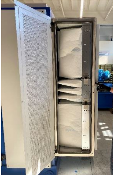
Remove the bolts and open the door
