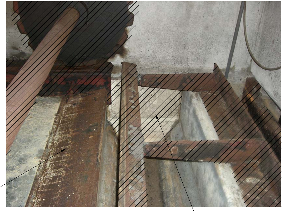
PHOTO 1 REMOVE TEMPORARY CONCRETE DIVIDER TO CONNECT TWS CHANNELS BETWEEN TANKS 3 & 4
